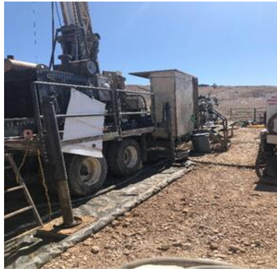
Figure 8-1: Truck Mounted Core Rig
