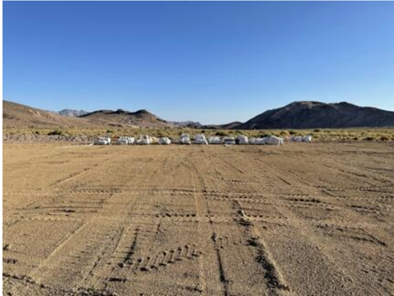
Figure 8-2: Laydown Yard and Sample Storage
